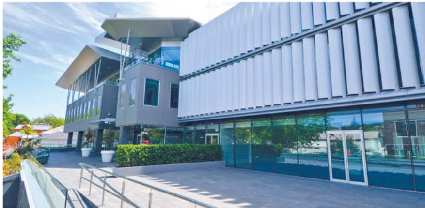
FULLY LEASED: Mansons TCLM's GHD Building
